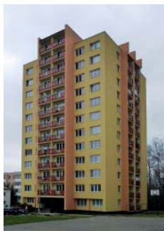
Fig. 1 Prefabricated house T 06 B-BTS (Prefabricated houses, 2010)
