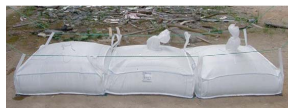
Fig. 16 Connecting three sealing bags side by side and their fixing in place with ropes
