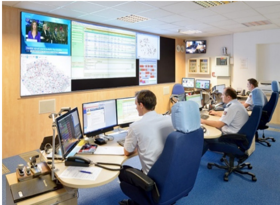
Fig. 5 Operation and information center (AV Media, 2019)
